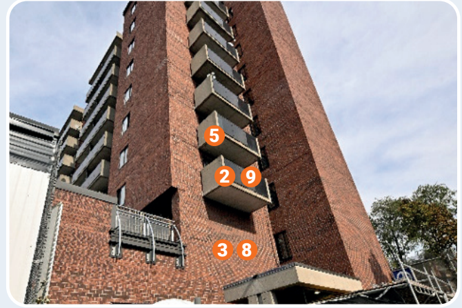
Façade overlooking Berri Street
