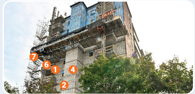
Façade overlooking Lajeunesse Street
