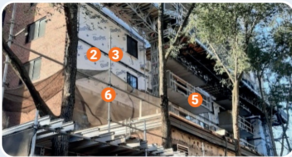
Façade overlooking the alley
